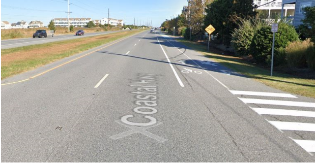
Figure 07A – Expanded shoulder for pedestrian/bicycle use – State of Delaware Coastal Hwy 1
