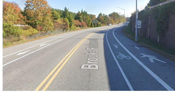
Figure 07B – Expanded shoulder for pedestrian/bicycle use – State of Maryland – Brooks Robinson Drive Pikesville, MD
